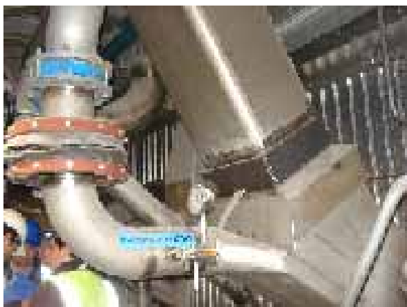
Detailed view of waste and air inlets
