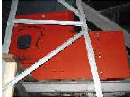
Rejects crushed to 5-20 cms before being fed to fuel preparation plant
